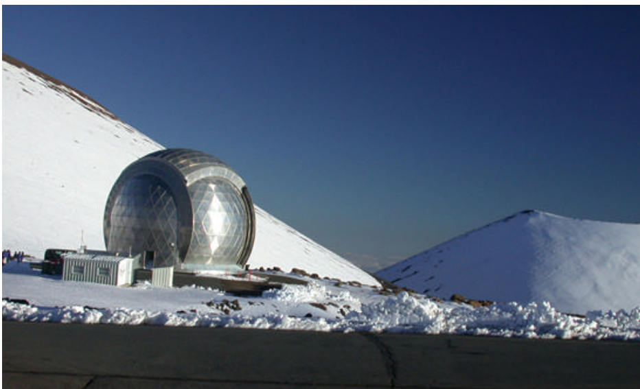
The CSO dome in the closed position.
